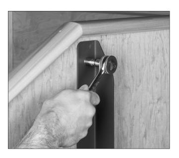
After the right and left handrails have been fully tightened, go back and fully tighten all of the uprights at the base.
