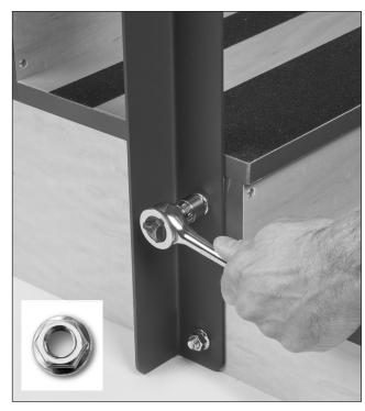
Once all the uprights are in place, it is important that you attach the rear handrail FIRST. Position the rear handrail on the outer side of the rear uprights and put the four (4) 1-1/4" Phillips head bolts through the wooden handrail and the steel uprights.
