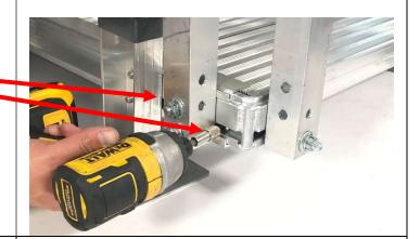
7. Once all straight and corner picket connections have been made and switchback bracket is secured to platform, fully tighten all leg and handrail nuts.
