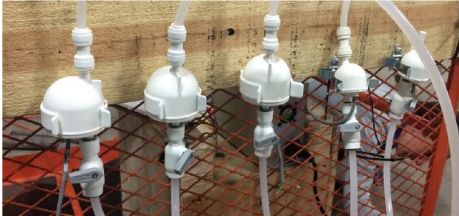
Figure 2-4: Example of Micro units with plumbing installed
