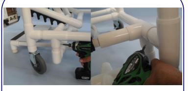
SECURE USING 1/2" RETAINING SCREWS AND PILOT HOLES AS REFERENCE..
