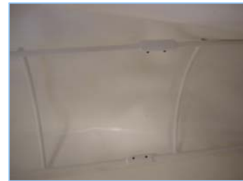
‘Side support tightened into place
