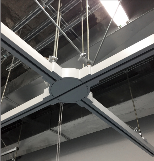
Location of 4 x 1/2" (114.3 mm) holes for the 1/2" (12.7 mm) threaded rods
