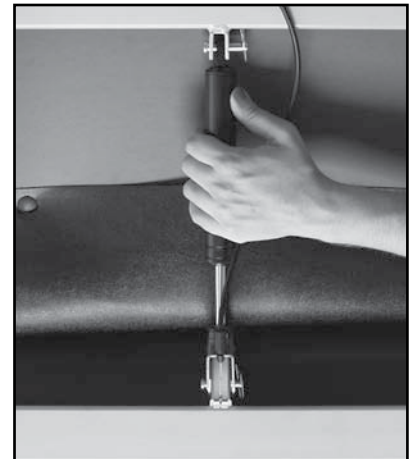
Adjusting Cable Tension 1
